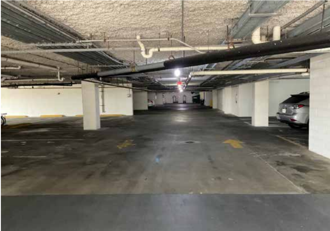
Parking Garage - Lobby Level
