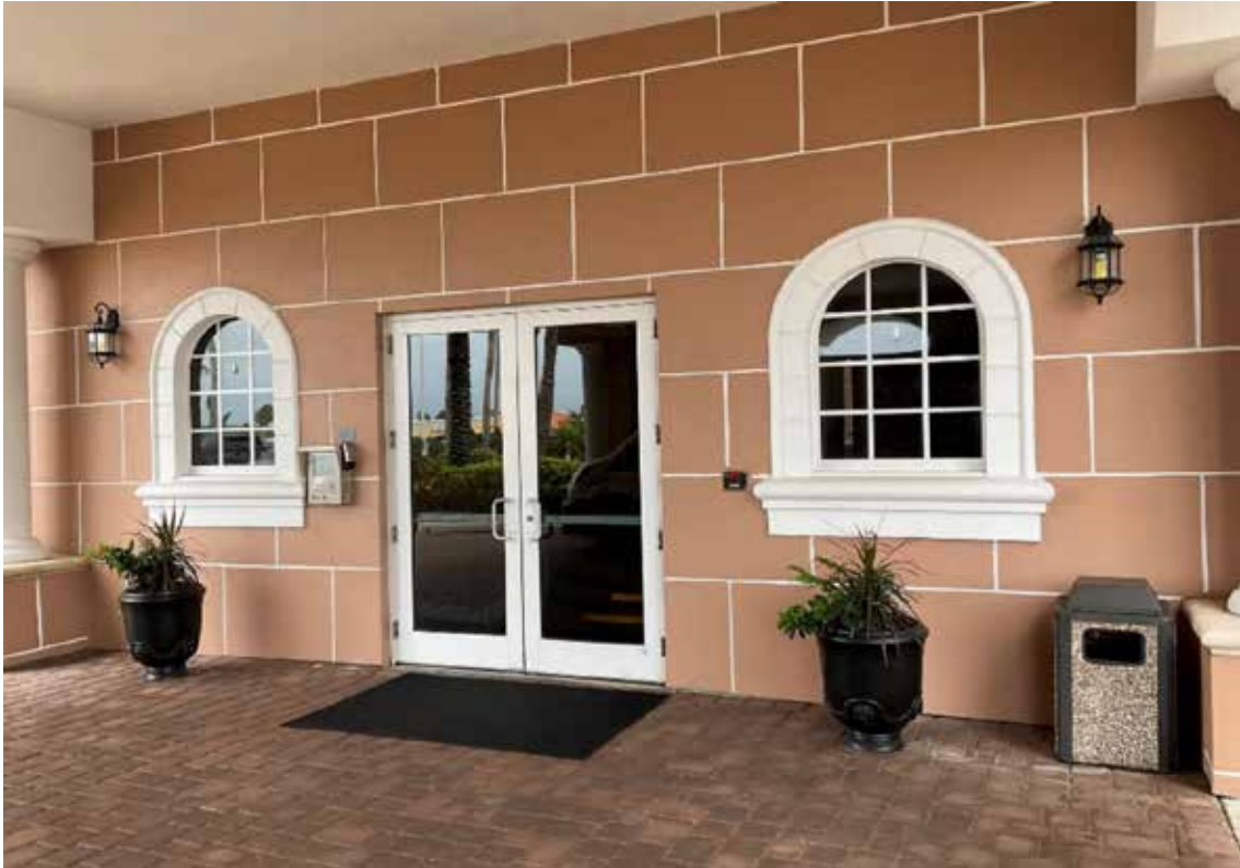
Main Lobby Entry
