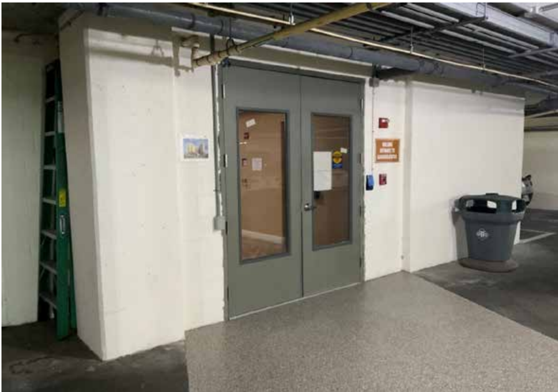
Door - Lobby Level Garage Access
