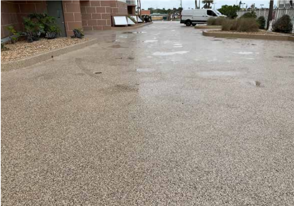
North Parking Deck w/Coating
