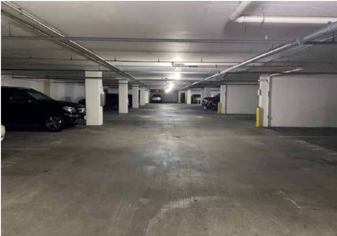
Parking Garage - Basement Level
