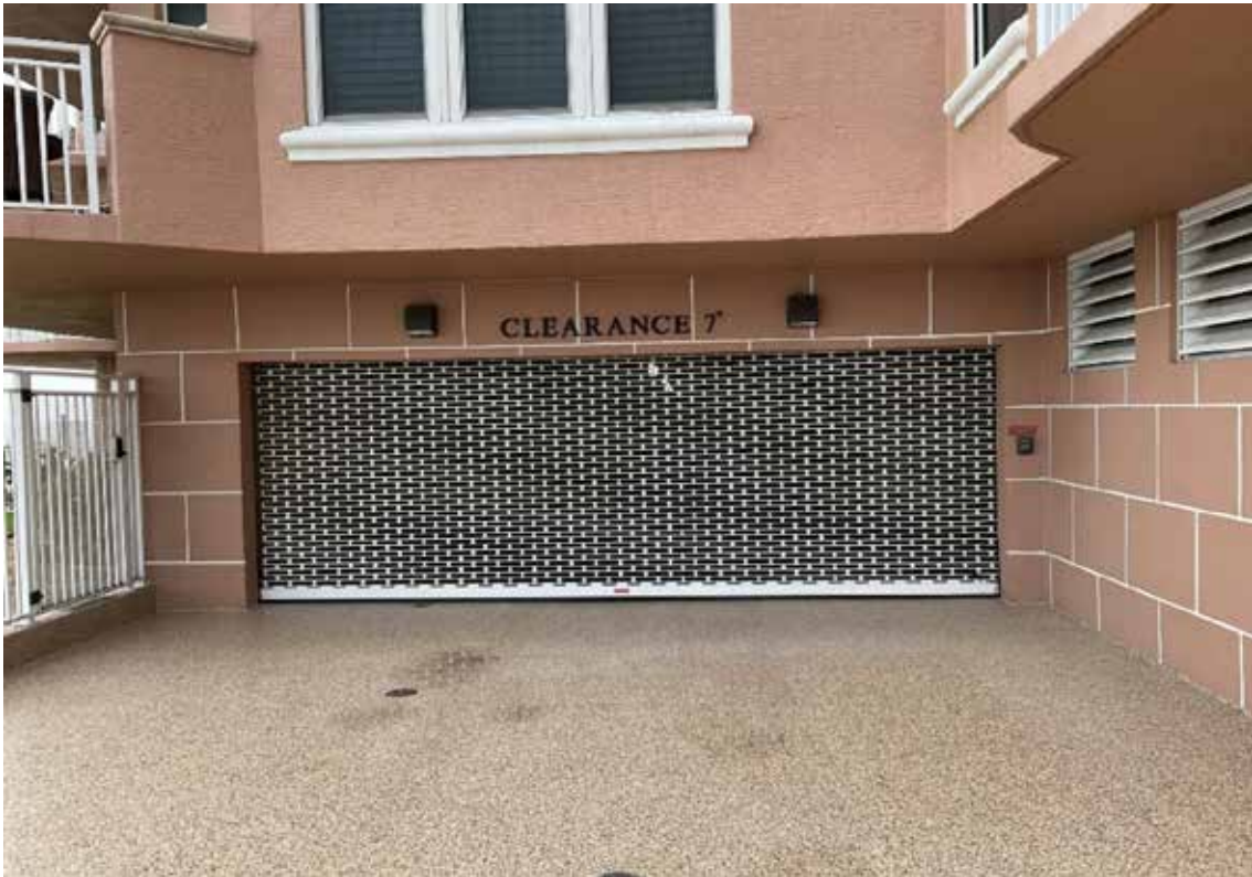
Garage Gate - Lobby Level
