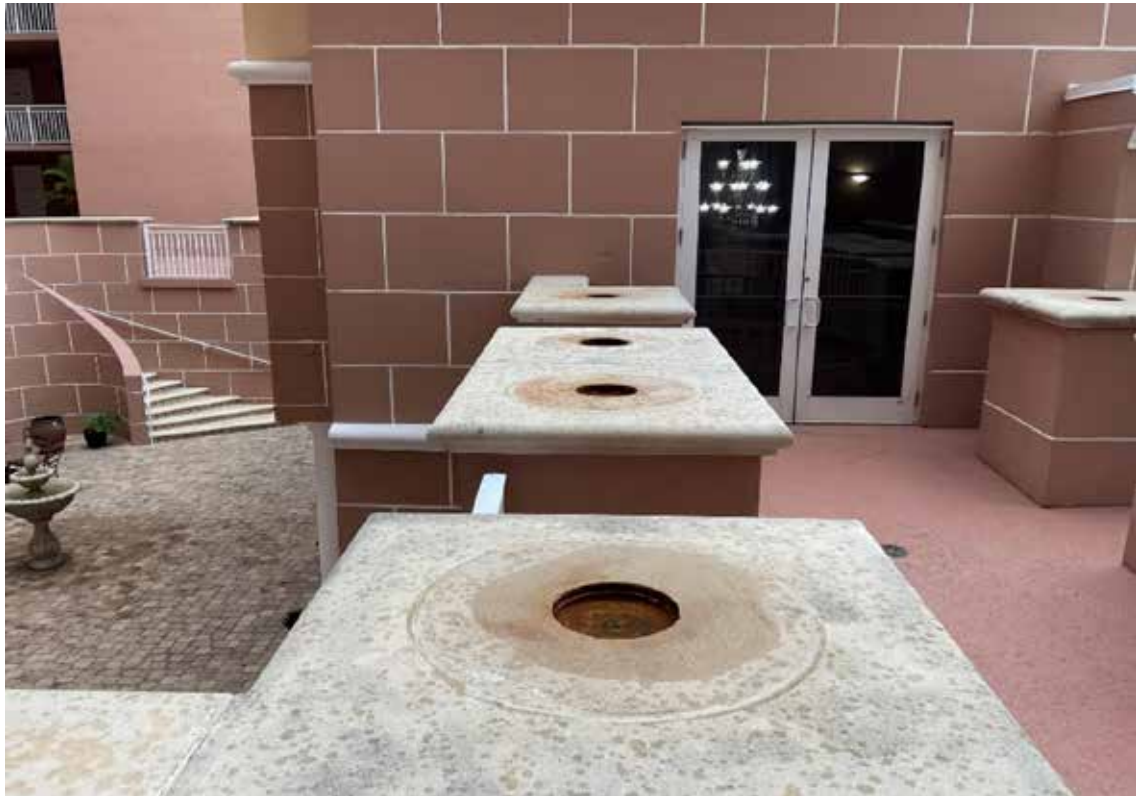
Level 2 (Old Pergola Location)
